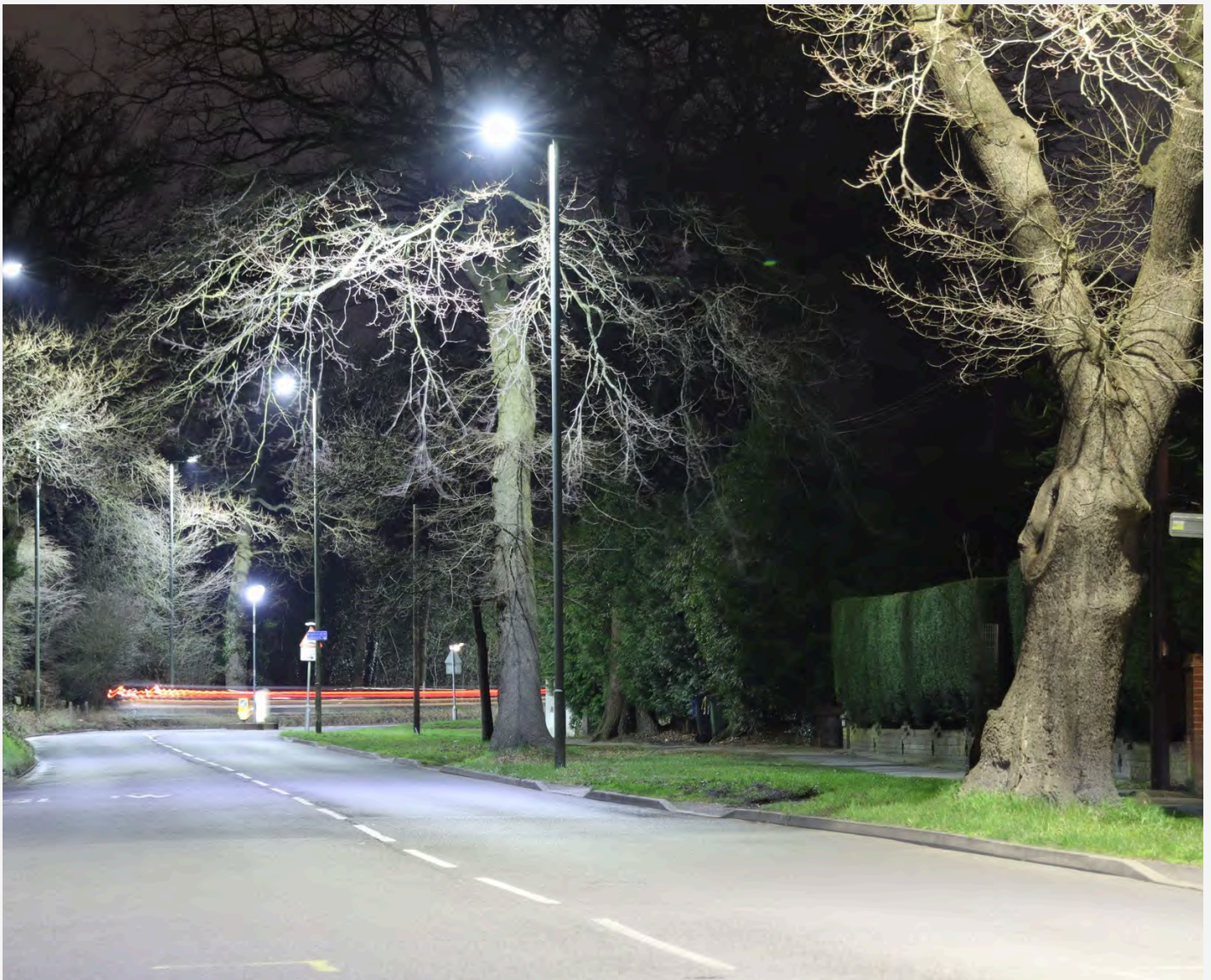
Photo above: Bromley LED streetlamp lighting upgrade
