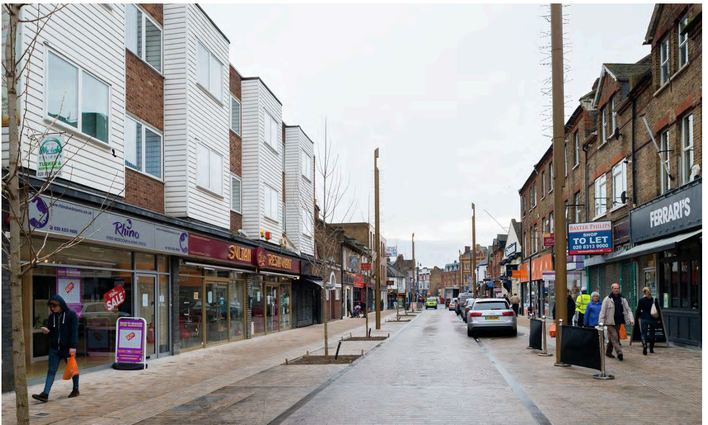
Photo above: East Street, Bromley, paving and street improvements
